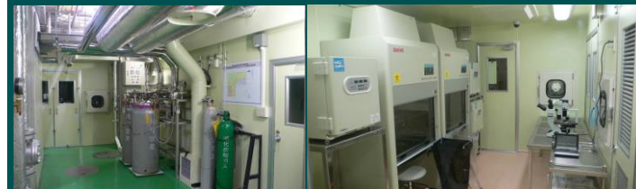
1. Entrance and Over view
